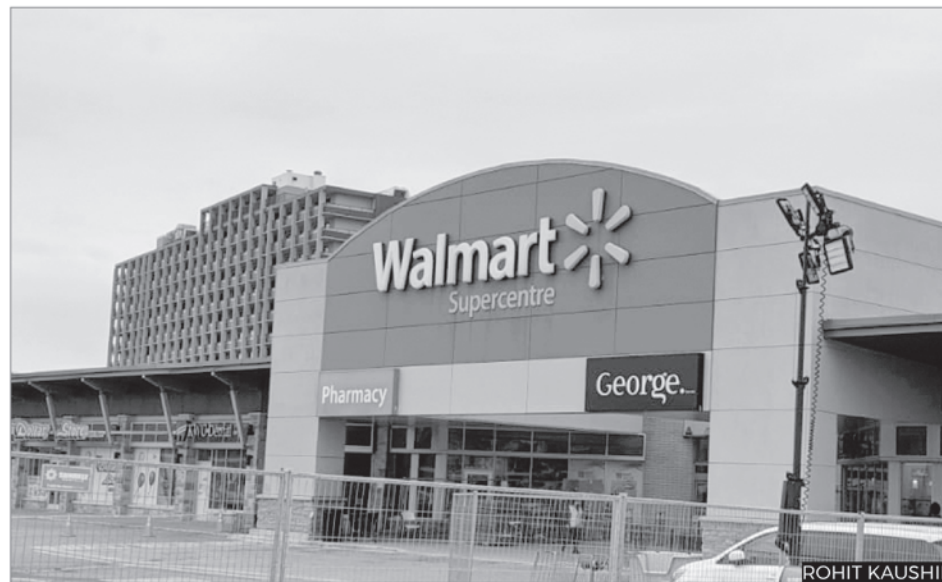
The early damage is estimated to be around $4 million per location.
